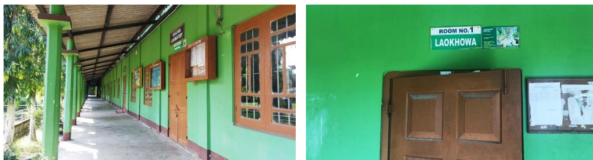
Photo 3: Classrooms of Kaliabor College.
